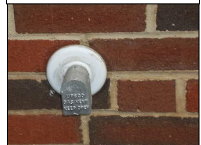
Sample Outside Vent for Indoor Gas Meter
