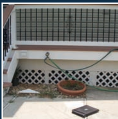
Deck Built Over Top of Pedestal Meter
