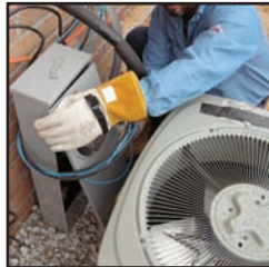
HVAC Unit in Front of Meter (Meter Installation and Removal Extremely Difficult)
