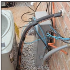
HVAC Unit in Front of Meter (Meter Installation and Removal Extremely Difficult)
